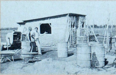
Another stack-sack home in the making.
